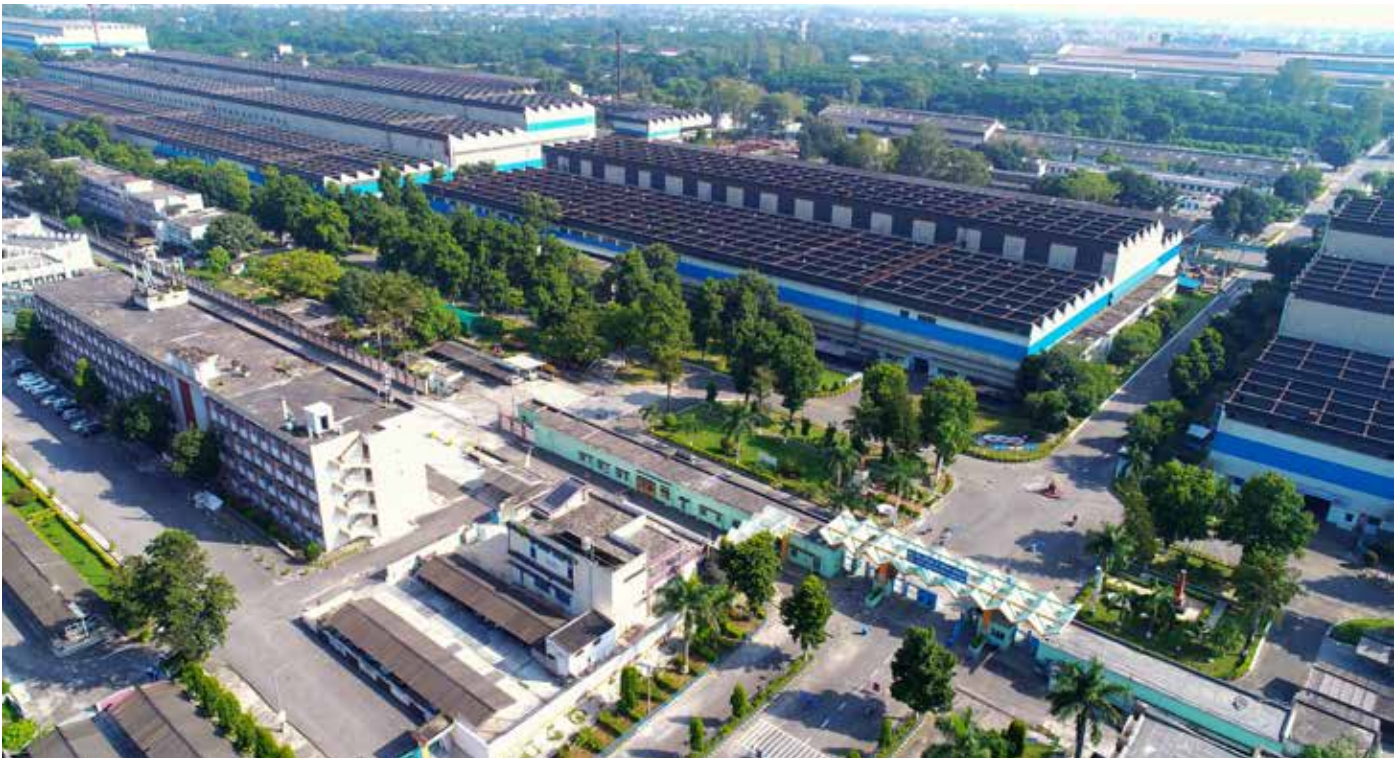
Heavy Electrical Equipment Plant (HEEP), BHEL - Haridwar
