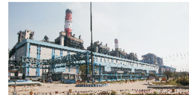
1x490 MW Power Project commissioned at Dadri
