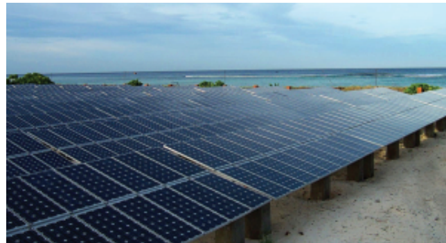
SPV Power Plant, Karnataka
