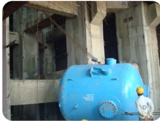
Flash tank being positioned below TG deck
