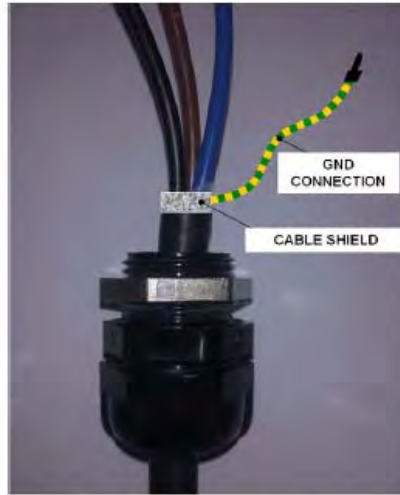
Figure 1 - Connection box shield connection
