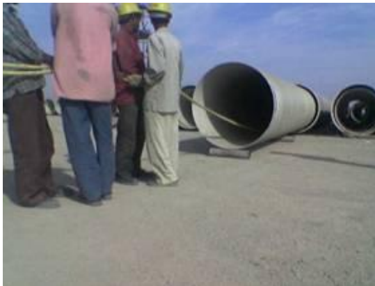
Nylon rope –with “C” Clamp Pulling Pipe on Roller Arrangement.
